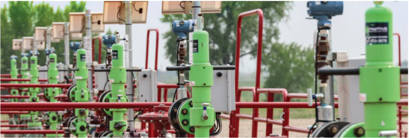
Figure 8: An example of Bayswater utilizing solar arrays to help power wellheads on a Colorado production site.
